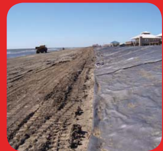
Grand Isle Beach Repair between Hurricanes Gustave and Ike, Laying Fabric, 2008
